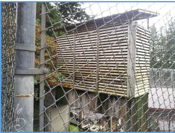
Figure: 16: The east side of the Hatchery
